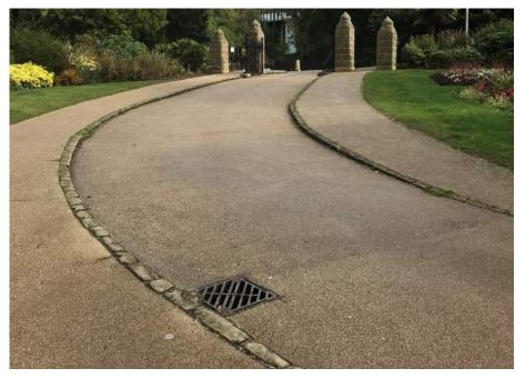
It is recommended that the existing gully cover is replaced with a cycle friendly gully grate.
