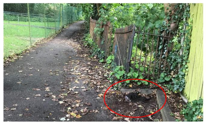
It is recommended that the existing gully and detritus buildup is cleared and that additional drainage provided if the existing system is no longer effective.
