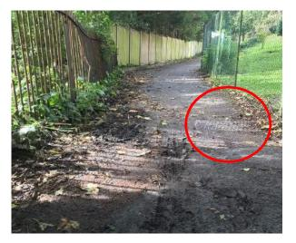
It is recommended that the utility covers are treated so that they provide a consistent surface finish and skidding resistance to the shared route surface.
