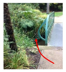
It is recommended that additional sections of extended parapet are provided at all bridges with adjacent gaps/steep drops into waterways.
